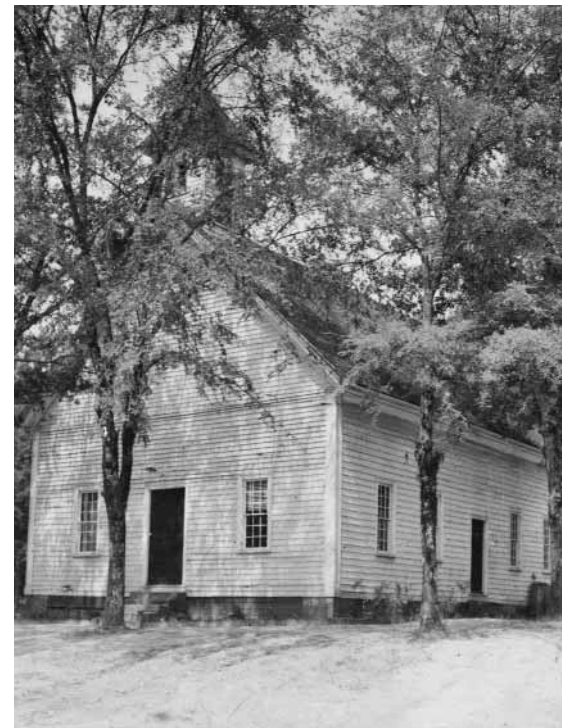
Clinton Methodist Church, circa 1935. Located on Dames Ferry Road and built circa 1821, this is reportedly the first Methodist church and the second church established in Jones County.
